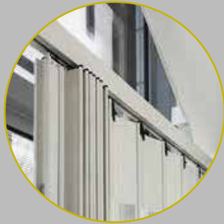
Guida superiore Top-hung track
